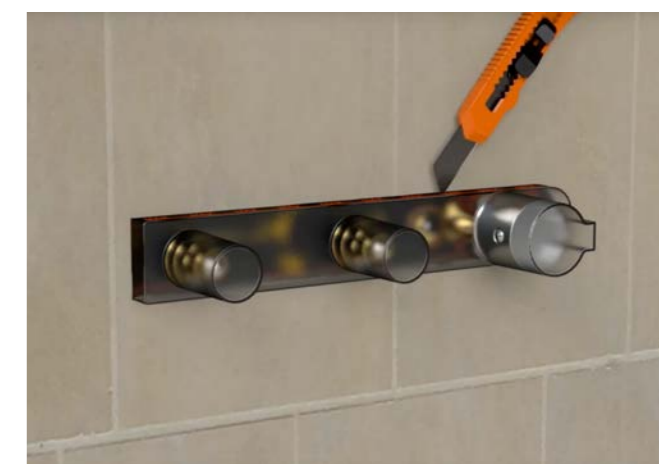
4. Once tiled it is easy to remove the protective case with a sharp blade
