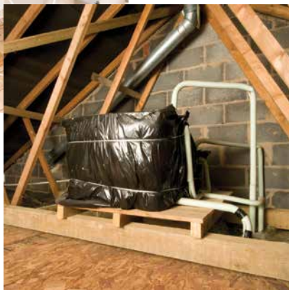
cold water tank installed in the loft
