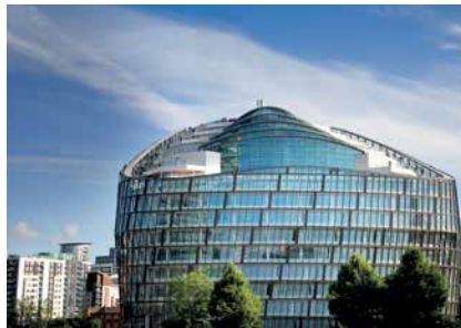
Co-operative Group Headquarters, UK
