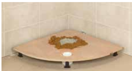
5. Mix bedding sand and cement (included in kit) on the Trayed Secret base.
