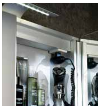
Shaver socket located at top of cabinet
