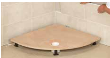
4. Finish tiling and use the Trayed Secret system as a working platform.
