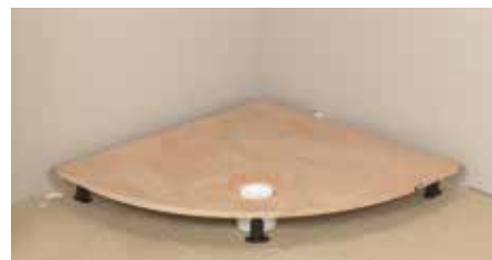
3. Place the Trayed Secret system into position. 3. Placez correctement le système Trayed Secret.
