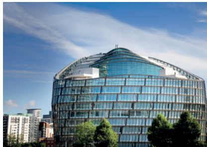
Co-operative Group Headquarters, UK
